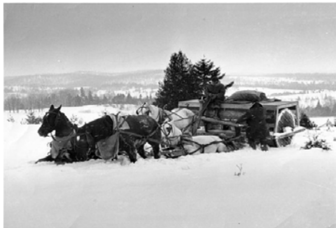
Snow roller circa 1941 in use in Vermont. The horses had winter calks on their shoes. A calk is a blunt projection that is often forged, welded or brazed on the shoe. The term may also refer to traction devices screwed into the bottom of a horseshoe called shoe studs or screw-in calks
